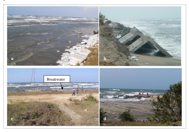
Figure 5. Shore protection measures installed at the 20<sup>th</sup> km. a,b,c. Breakwater made with panels of reinforced concrete (Photos taken in April, 2011 by author). d Sandbags installed to trap sediment (Photo taken from the road toward the northeast on May 28<sup>th</sup>, 2014 by Cristóbal Pizarro).
