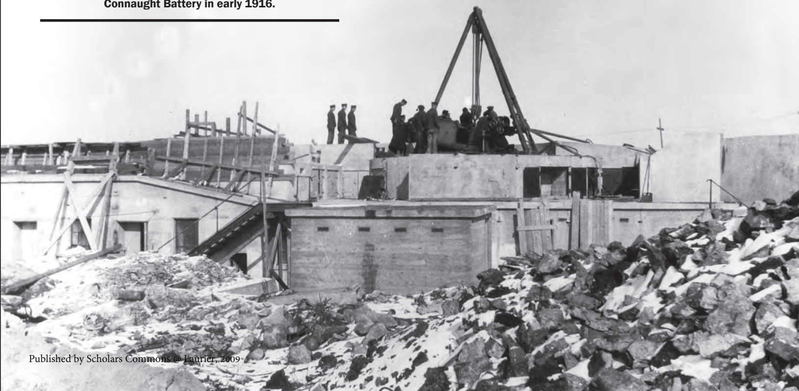
Workmen mount a 4.7-inch Quick-Fire gun at Connaught Battery in early 1916.
