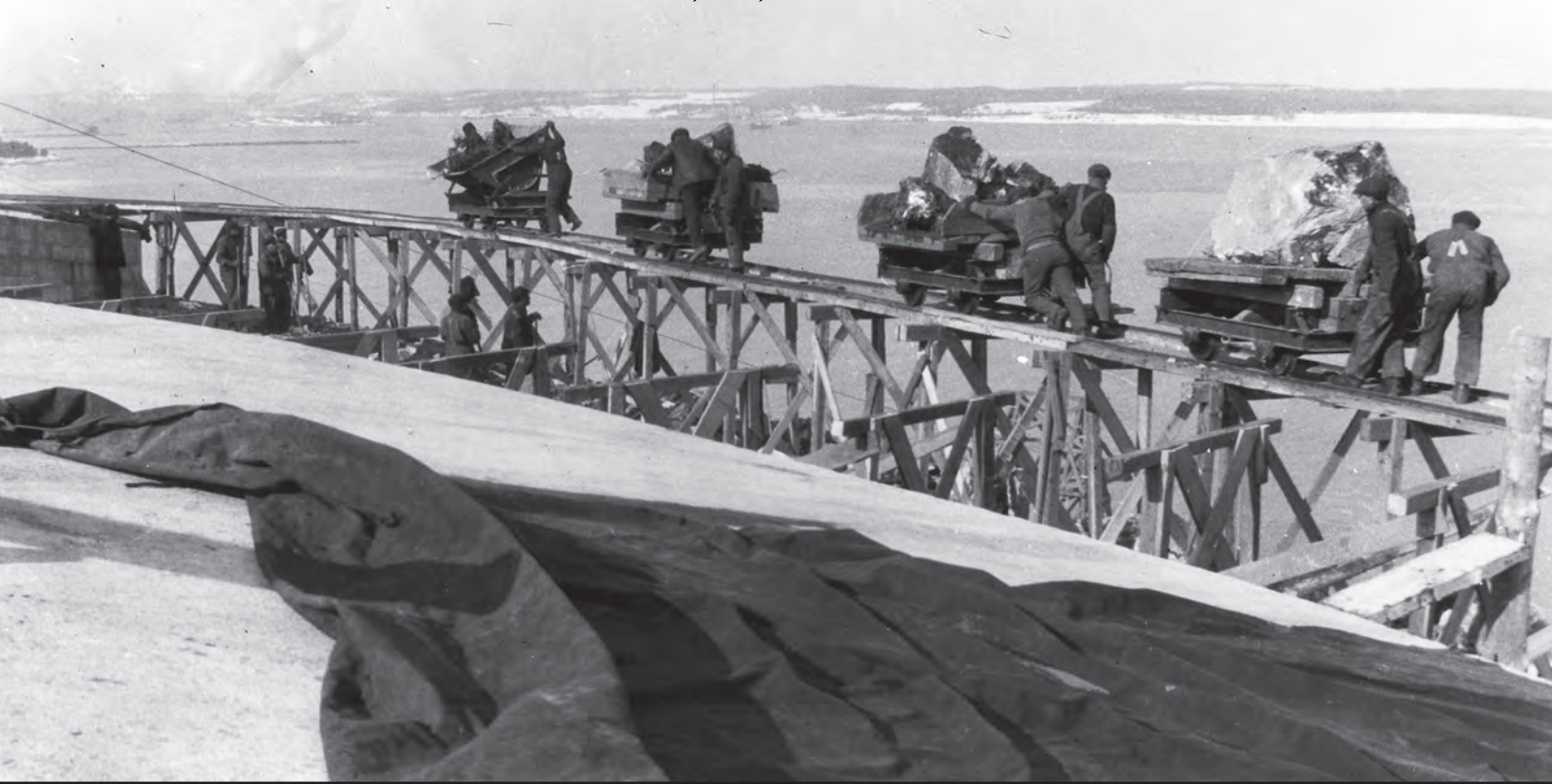
Dumping granite fill on the harbourward face of Connaught Battery from the light rail system that assisted construction. This photo was likely taken in early 1916.
