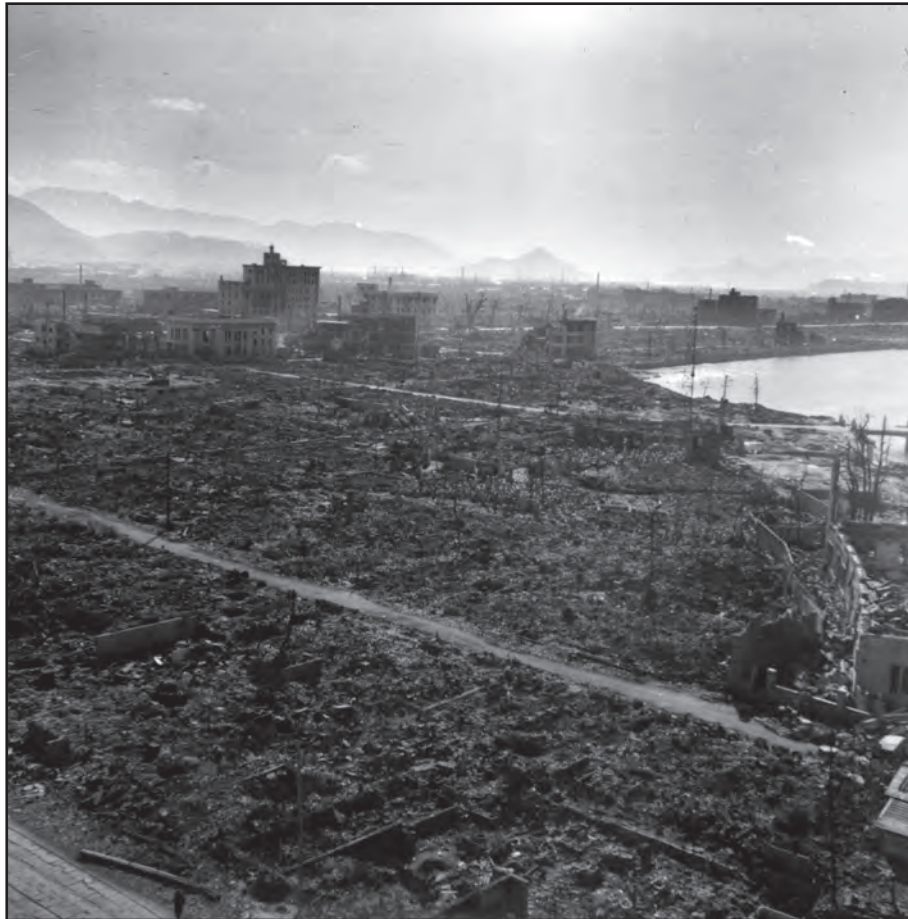
Hiroshima – A general view looking across the centre of damage. Some framed buildings quite near the centre remained standing. The foreground illustrates the remains of Japanese dwellings, razed to the ground.
