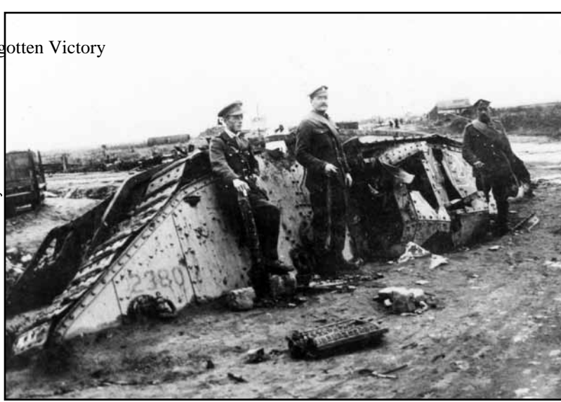
CWM 19750085-010 Destroyed Tank
