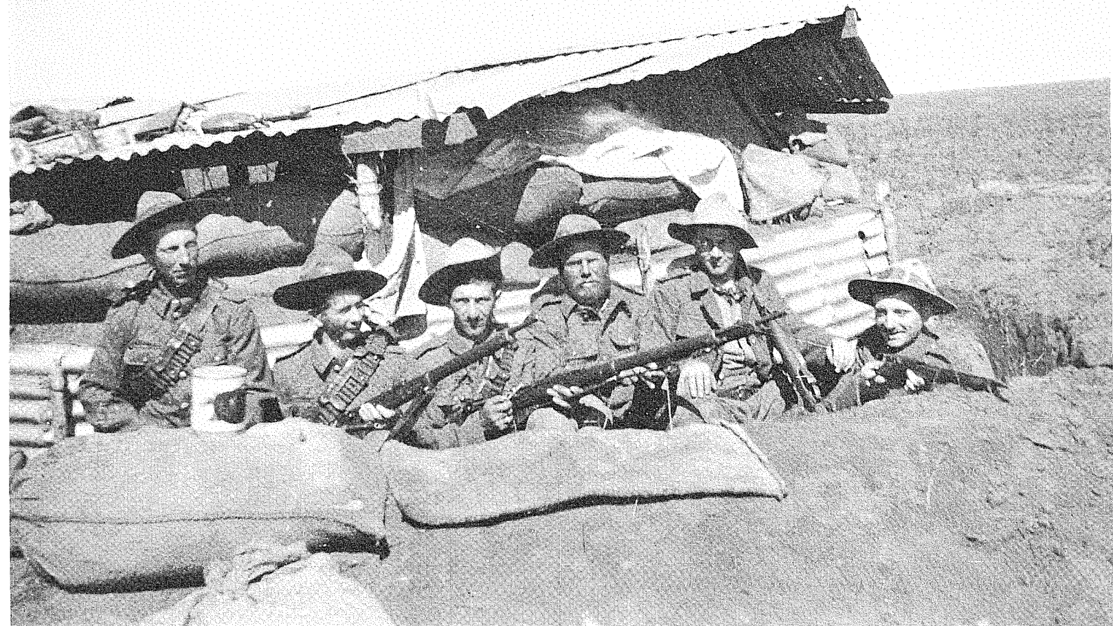
No inscription. An obviously staged photo providing a good view of a blockhouse and its defenders. Corrugated iron was common as a building materiel in South Africa, as it was to be later in the First World War.
