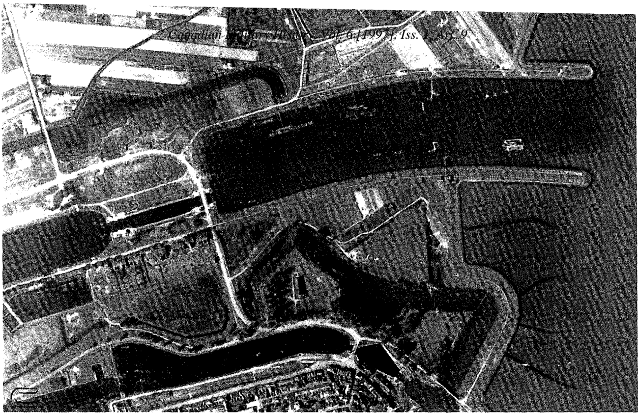
Above: The outer harbour of Ternuezen filled with shipping on 13 September.
