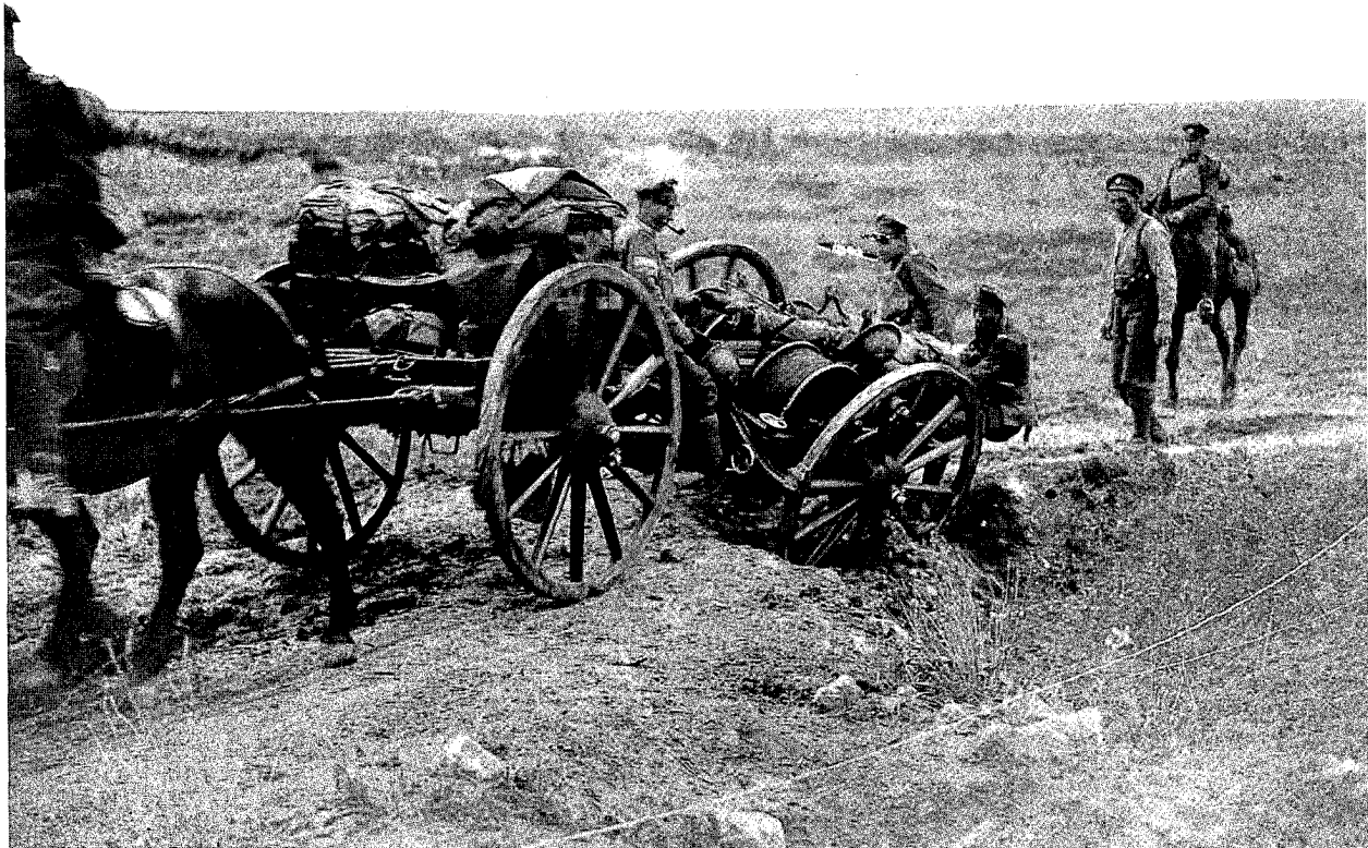
Canadian Signal Section laying cable during the advance east of Arras, September 1918.
