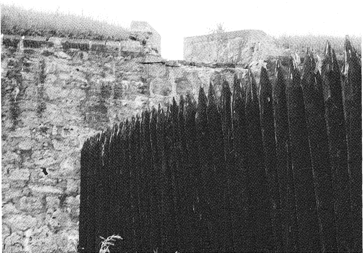
Looking up over the pallisades at the northeast bastion from the trench.
