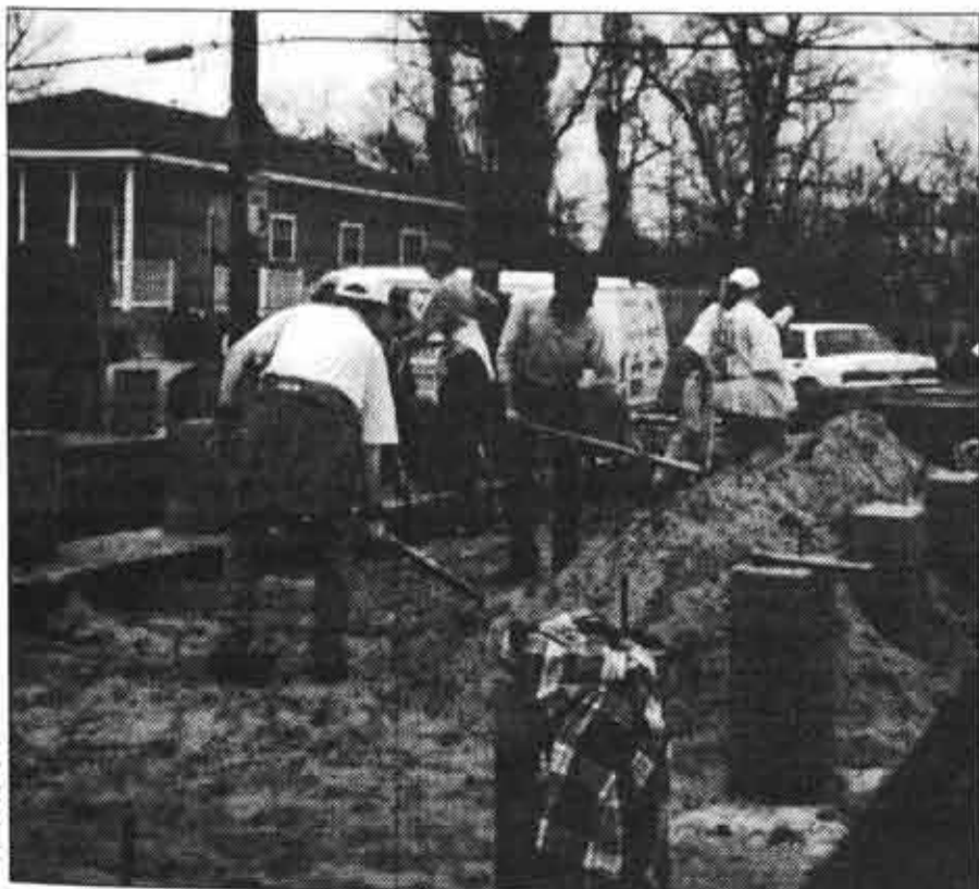
Students help out Habitat for Humanity by digging foundations.
