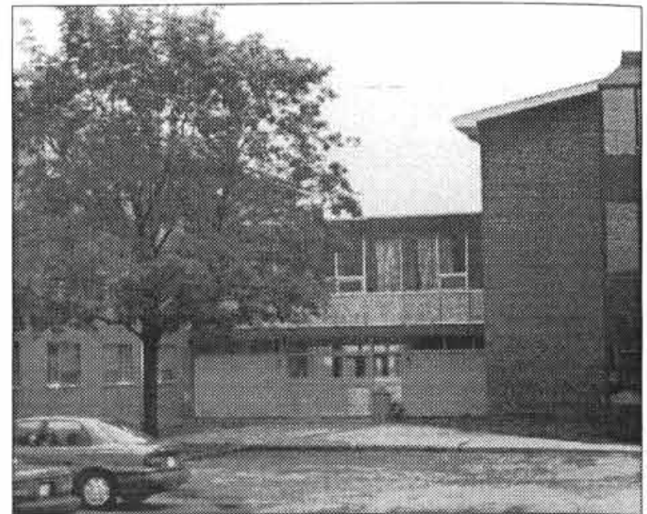
Laurier's Willison Hall underwent substantial renovations this summer to repair several major problem areas.
