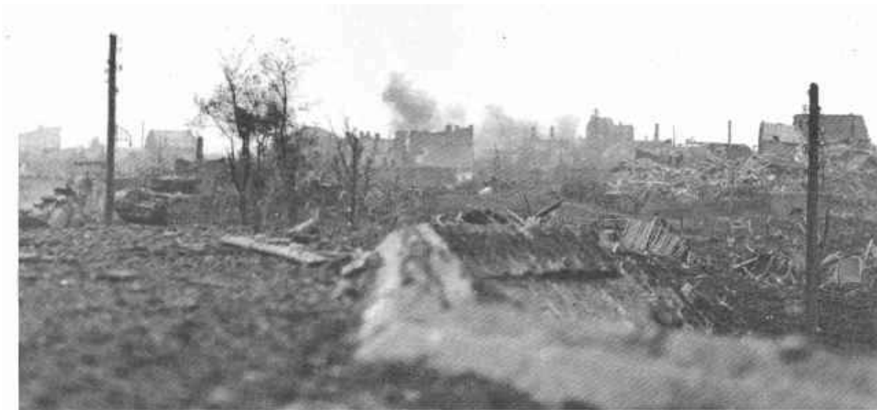
Artillery shells landing in Breskens, 22 October 1944. Note the Churchill AVKE at the left side of the photo. Photo by Donald I. Grant, NAC PA 138437
