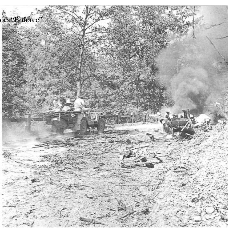
A Jeep Ambulance of 9 Field Ambulance passes the wreck of a German lorry knocked out by West Nova mortar fire south of Anzi after a German engineer detail was caught in the act of blowing a bridge. (NACPA 193390)
