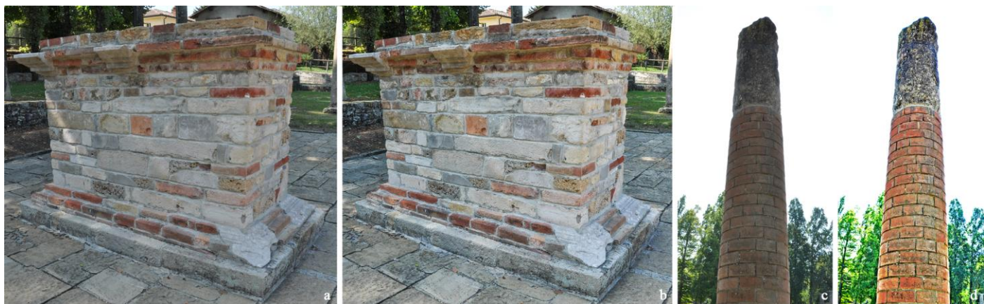
Figure 2. Examples of correction of illumination conditions. In (a) and (c), original images acquired using an uncalibrated Nikon D90 camera with variable focal length. In (b), elimination of highlights; in (d), correction of a backlight.
