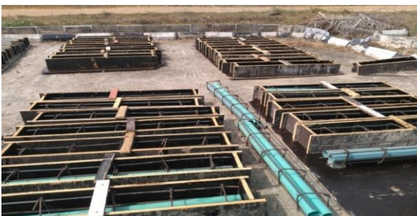
Fig. 6: Beam formwork with and without PVC pipes
