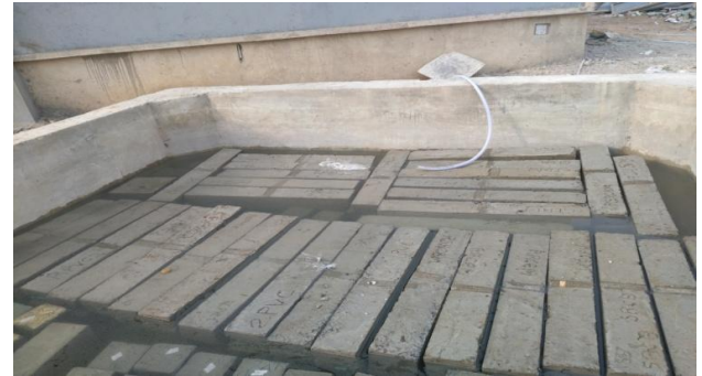
Fig. 8: Curing of beams in a curing tank
