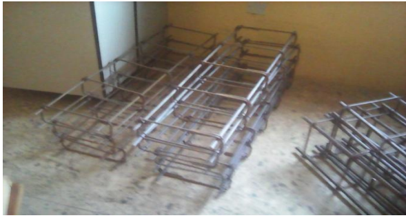
Fig. 4: Reinforcement cage with shear links
