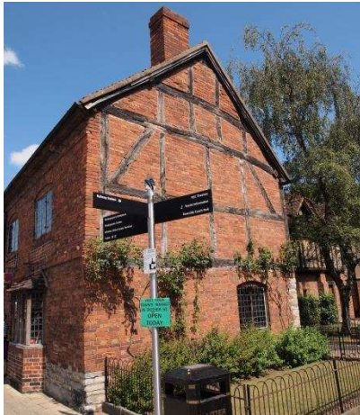
Figure 1 Half-timber frame with brick infill
