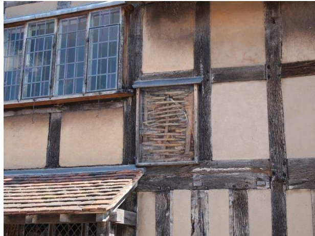
Figure 2 Half-timber frame with wattle and daub infill
