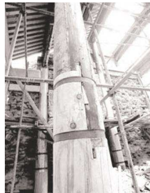
Figure 8 Partial replacement repair in Daibei Temple (1550), China [4]
