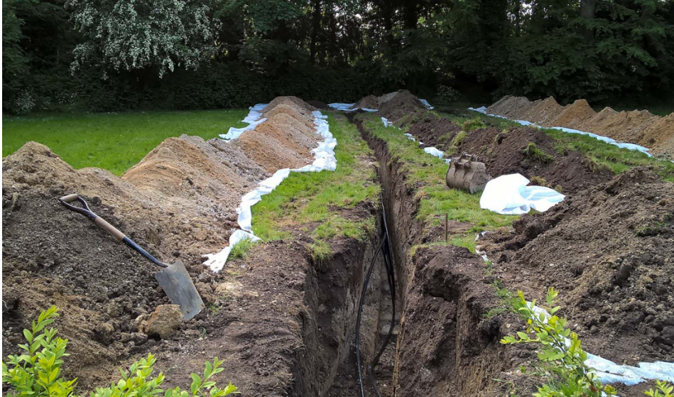
453 Figure 10 - Photo of ground loop excavation.
