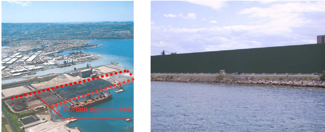
Fig. 5.3: Disposition of the curtain on coal terminal and the new curtain to prevent dust spreading (2004)
