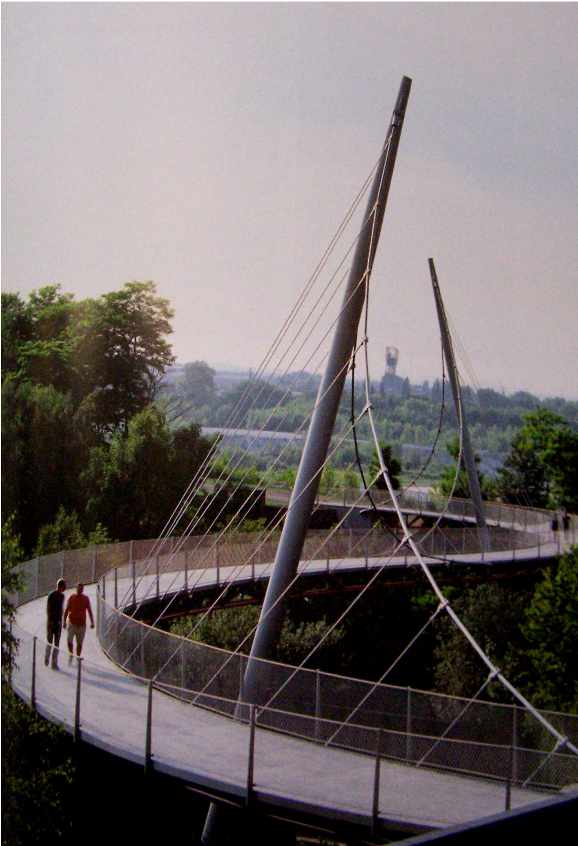
130 . Footbridge across the Gahlesche Strasse, Jorg Schlaich, Bochum, 2003
