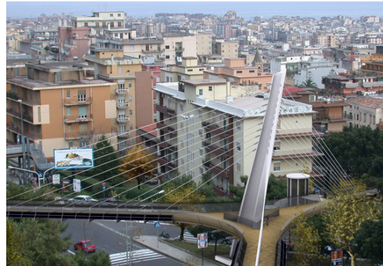
49. Footbridge in the University Cittadel
