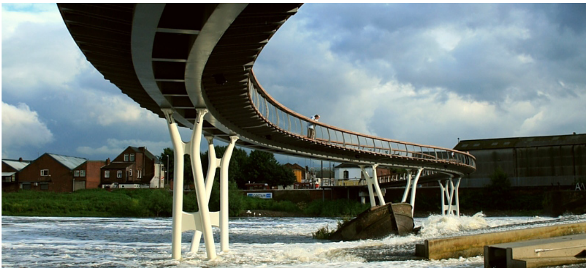
132. Castleford Bridge, McDowell+Benedetti, Castleford (UK), 2008
