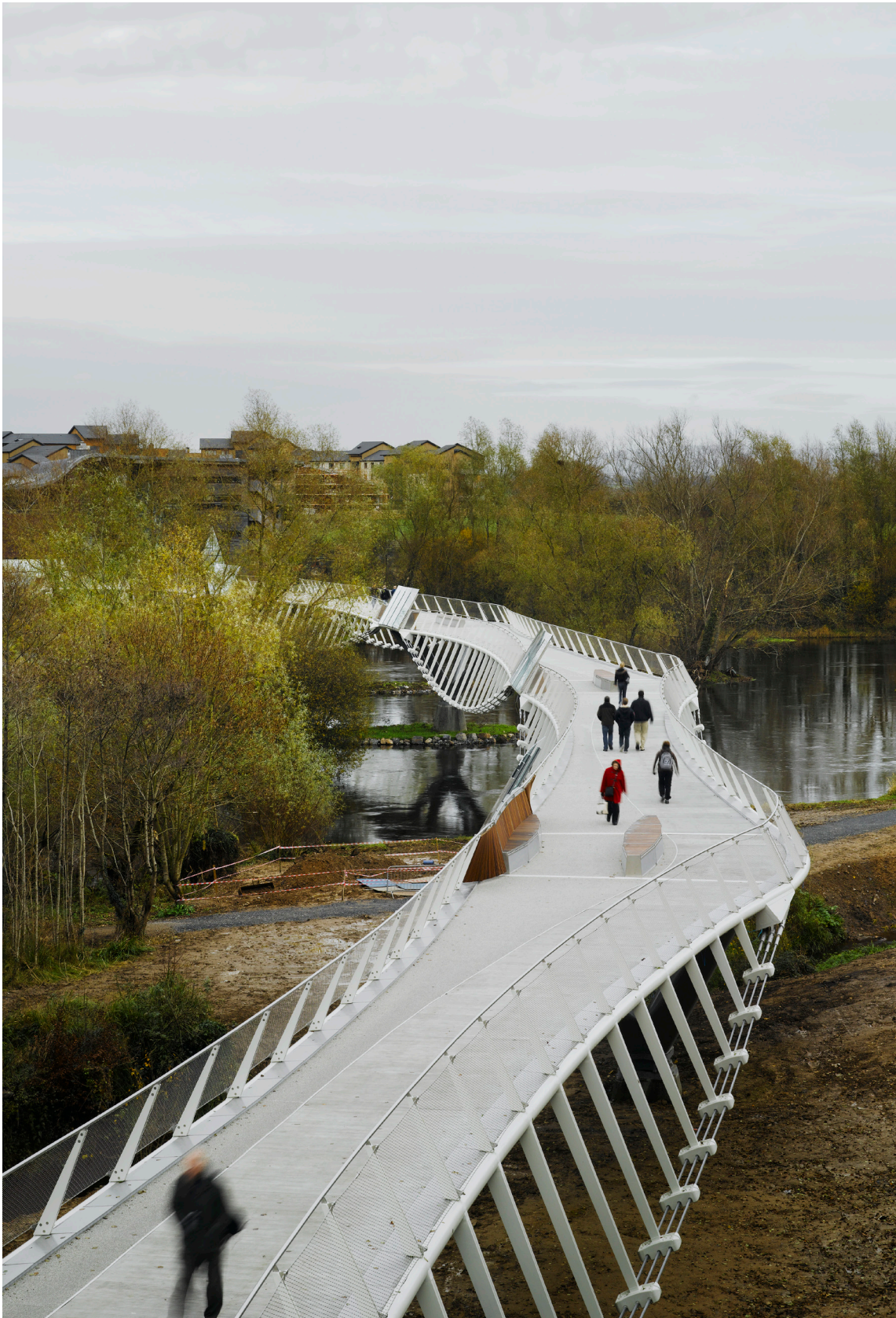
83. Limerick Living Bridge, Wilkinson&Eyre, Limerik, 2007
