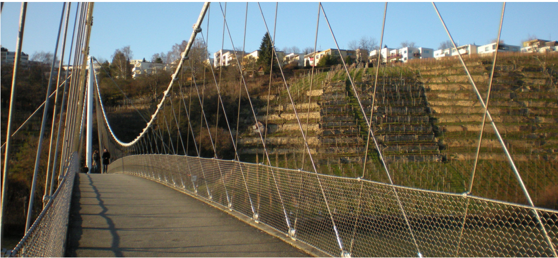
158. Footbridge on the River Neckar, Jorg Schlaich, Stuttgart, 1988
