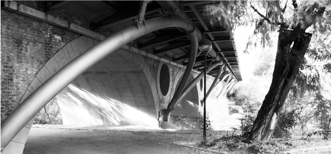
52. Borgo Tossignano Footbridge, Progeest, Bologna, 2005
