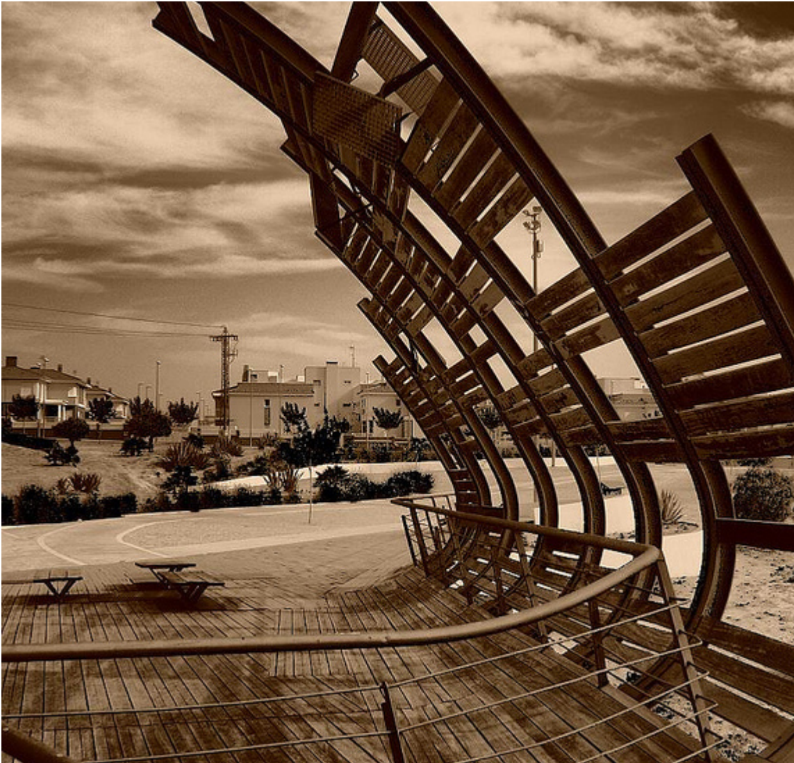
182. Footbridge, Carme Pinos, Petrer, Barcelona, 1991
