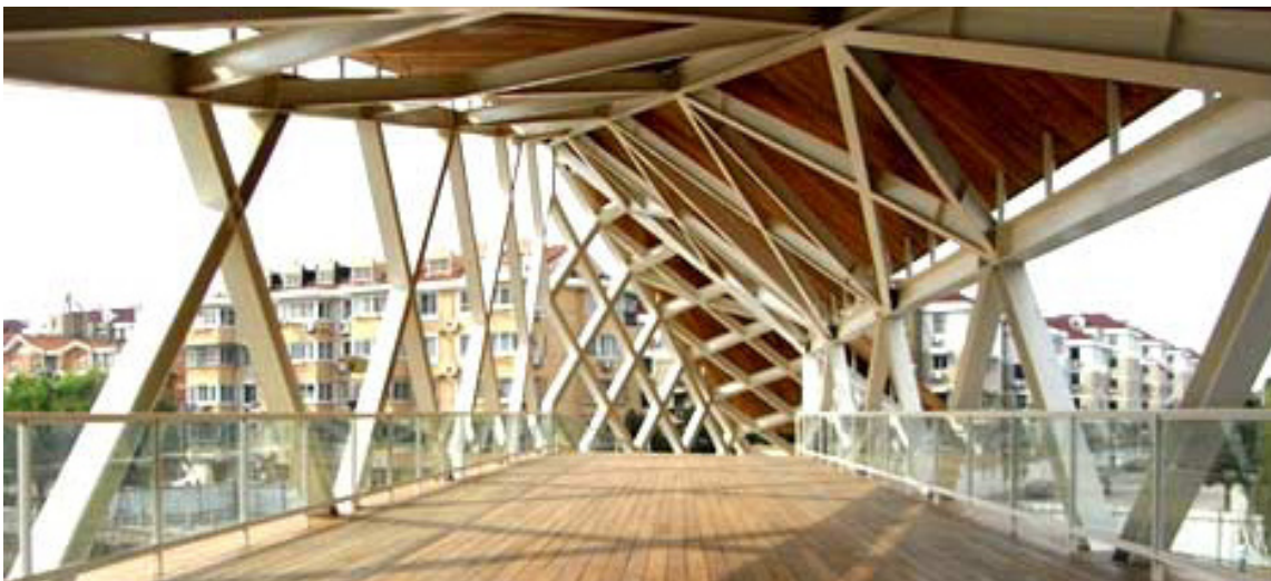
183. Footbridge, CA-DESIGN, Shanghai, 2009
