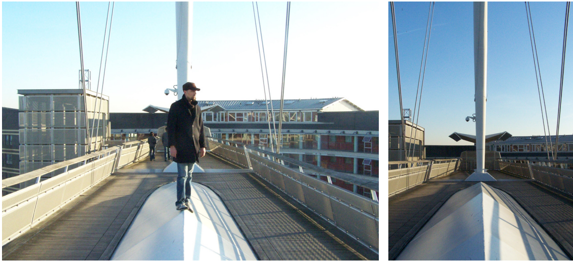
147. Royal Victoria Dock Bridge, Lifschutz Davidson Sandilands, London, 1998
