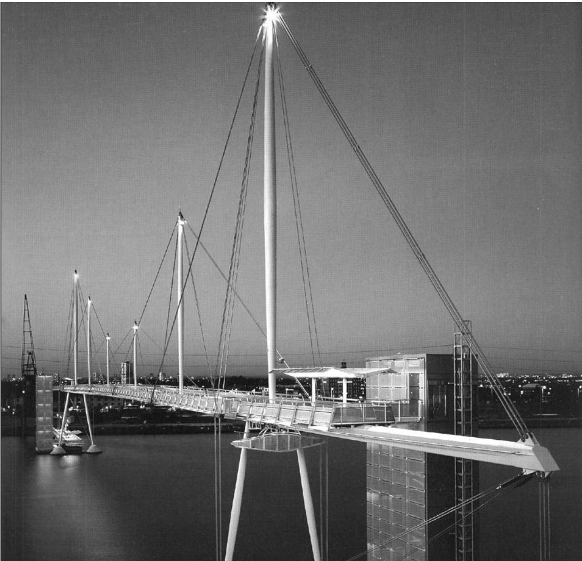
146. Royal Victoria Dock Bridge, Lifschutz Davidson Sandilands, London, 1998
