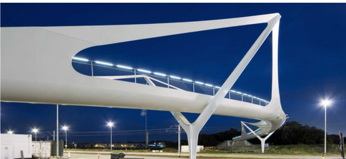
140. Knokke Footbridge, Ney&Partners, Belgium, 2007
