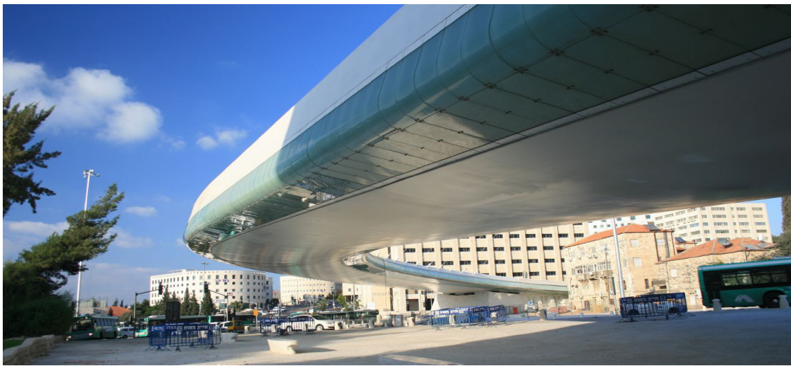
105. Chords Bridge, Santiago Calatrava, Jerusalem, 2009
