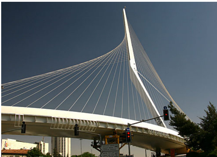
116. Chords Bridge, Santiago Calatrava, Jerusalem, 2009
