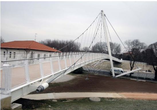
41. Footbridge across Via Venezia, Eng. Vitaliani
