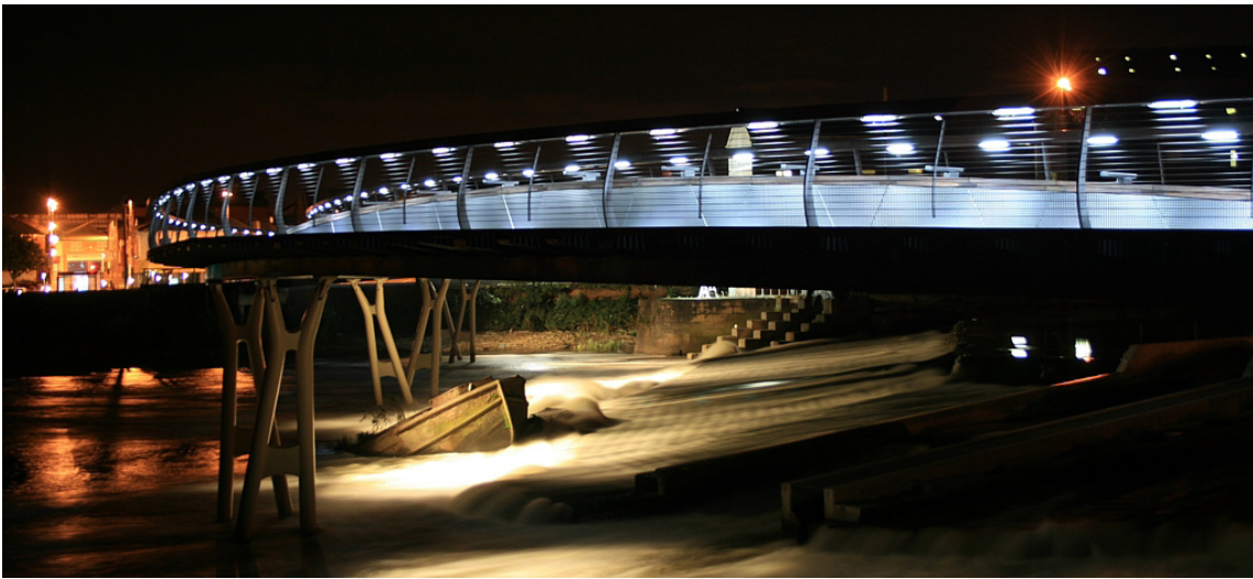
169. Castleford Bridge, McDowell+Benedetti, Castleford (UK), 2008
