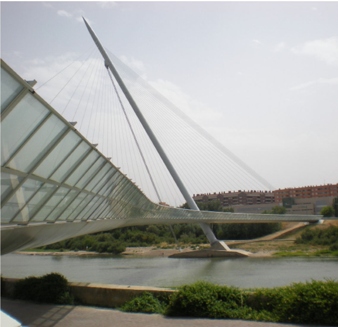
185. Expo Footbridge, Javier Manterola, Zaragoza, 2008
