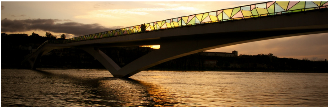
72. Pedro e Inês Footbridge, Adão Fonseca e Cecil Balmond, Coimbra, 2005
