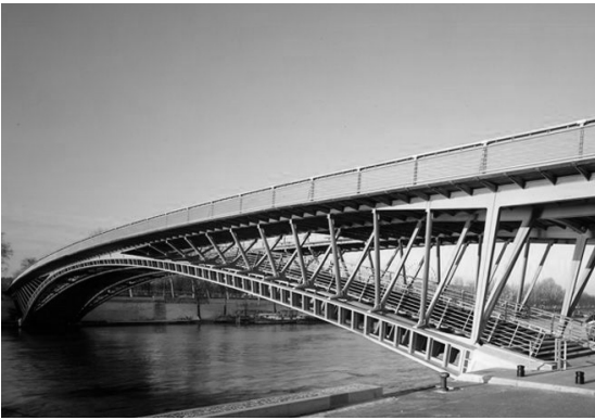
29. Solferino Footbridge, Marc Miram, Paris (1992-1999)
