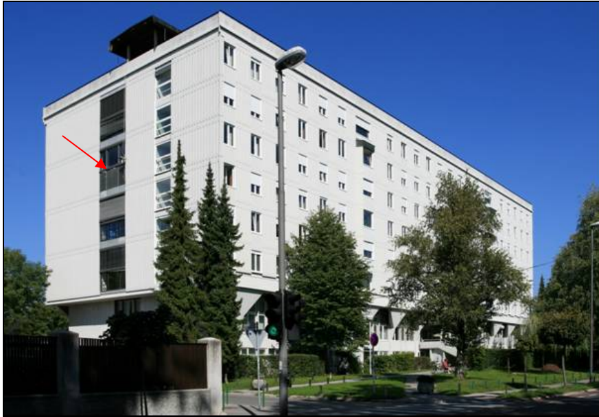
Fig 8: Test room, UL FGG, KSKE
