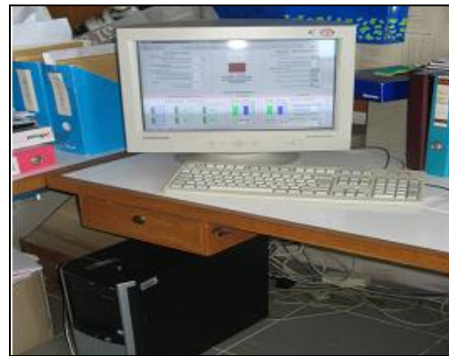
Fig 19: Building management system, software
