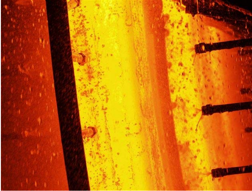
Figure 6.16: Spray systems in the Štore Steel billet caster.
