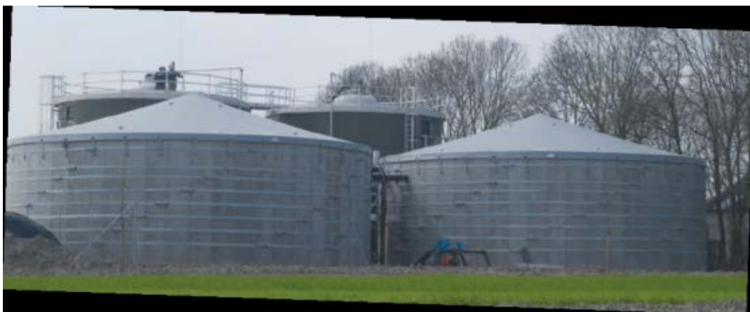
Figure 70: Manure is digested in on farm facilities into gas and digestate ( http://edepot.wur.nl/28917 )
