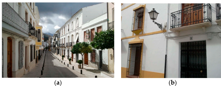
Figure 19. (a) General overview of the street; (b) Details of the lamp post installation.
