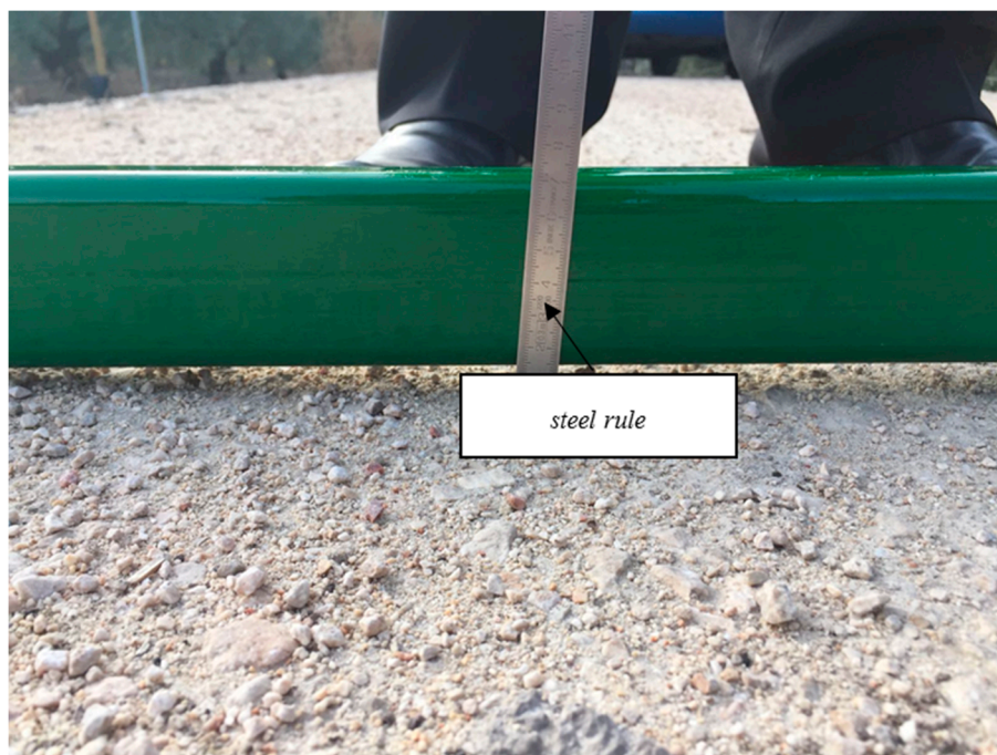
Figure 4. Rut depth measurement manually with straight edge and steel rule.
