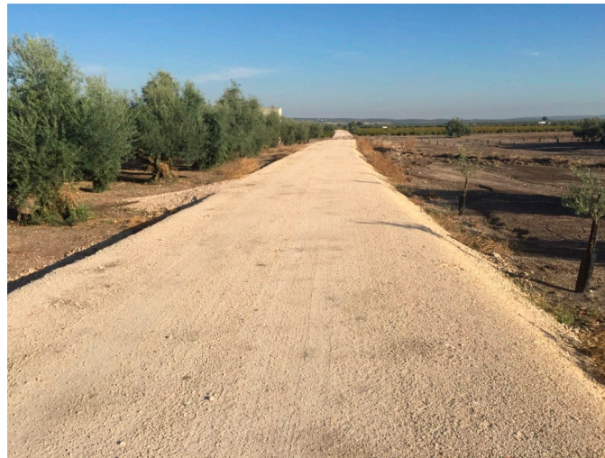
Figure 2. Section III of experimental unpaved rural road.
