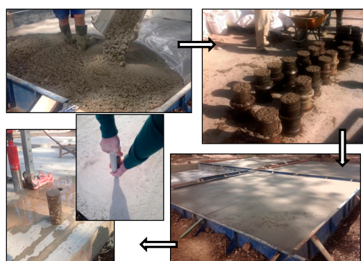
Figure 2. Slab execution, specimens cast and core extraction and non-destructive test.
