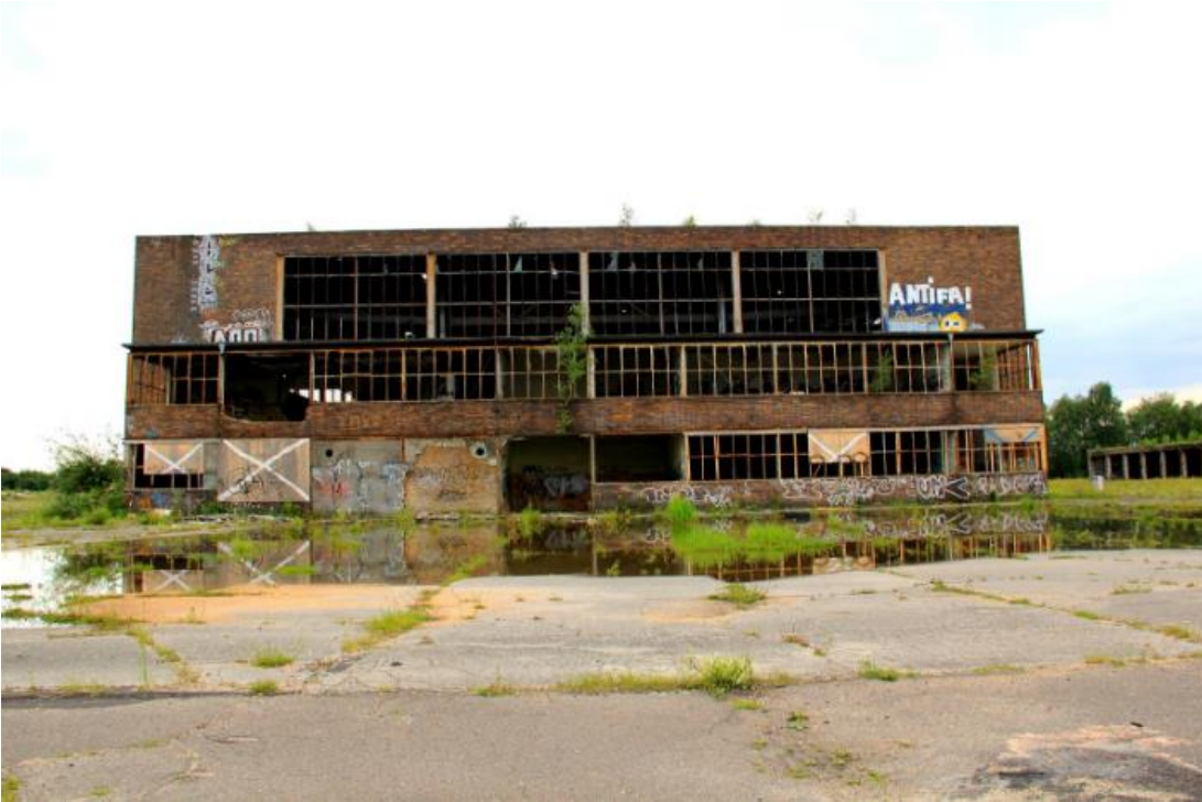
Fig. 5. Oranienburg Airfield before renovation
