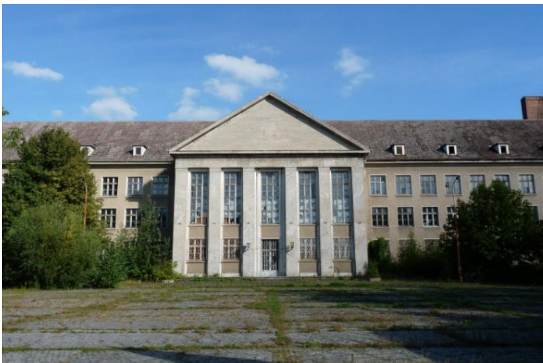
Fig. 4. Soviet Military Administration Headquarters in Karlhorst before renovation Source: Ciarán Fahey, 2010. Reproduced with permission of the author
