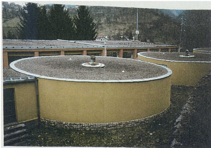
↕ A view of Stupari water treatment facilities
