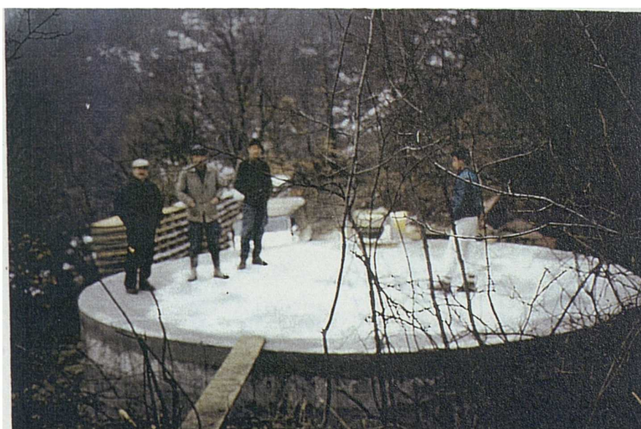
↑ The water pressure tank under construction in 1996
