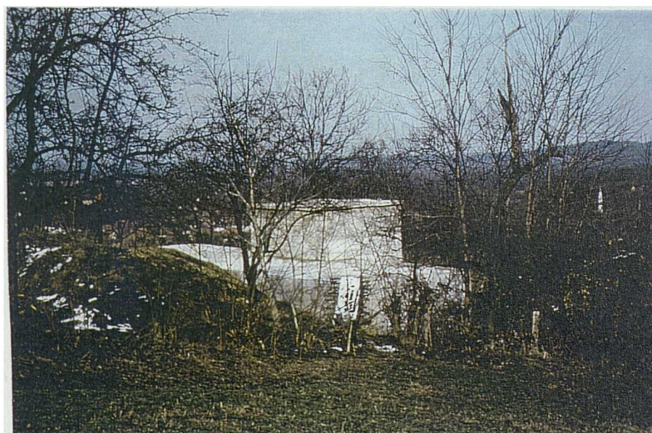
↕ The water tank with a capacity of 300 m 3
