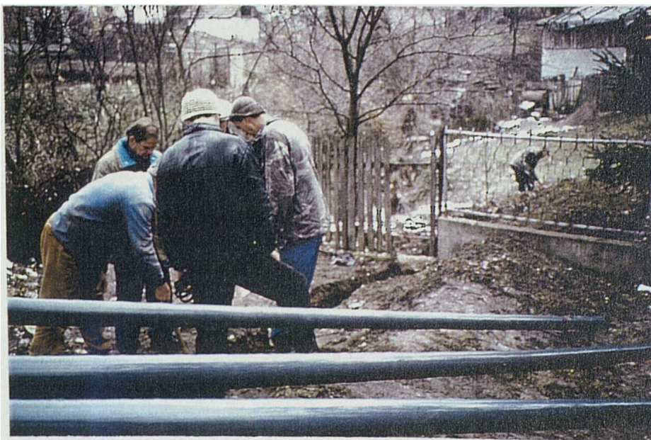
↑ The pipe laying under way in 1996
