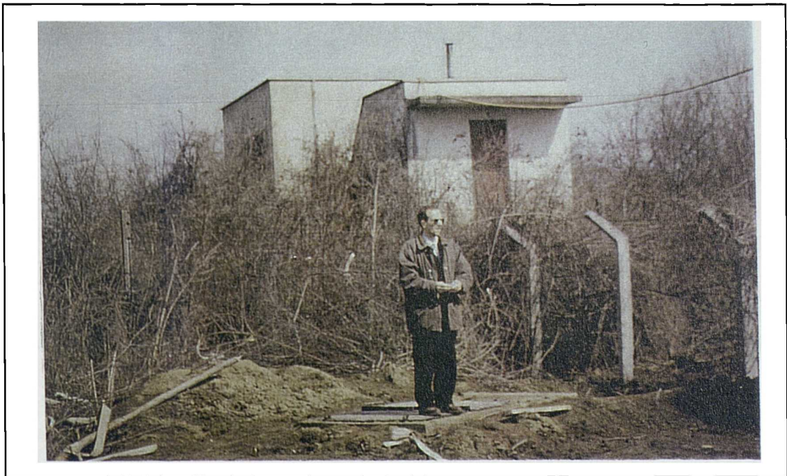
Figure 8.3: The Tojšići Water Supply's borehole and pumping station (Enver Agić is standing on the borehole) (Source: Author)
