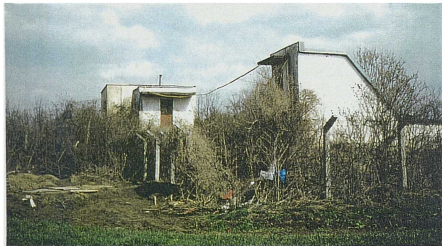
↑↓ Tojšići pumping station
