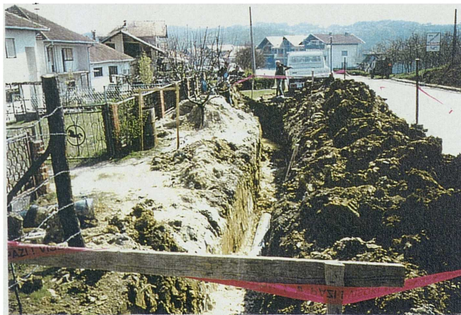
↕ The water pipe laying is in progress
