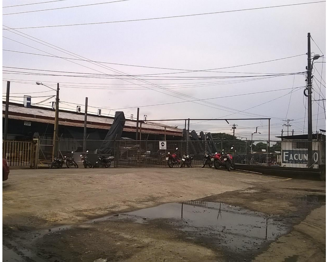
ECUAVEGETAL S.A. (Facundo)
