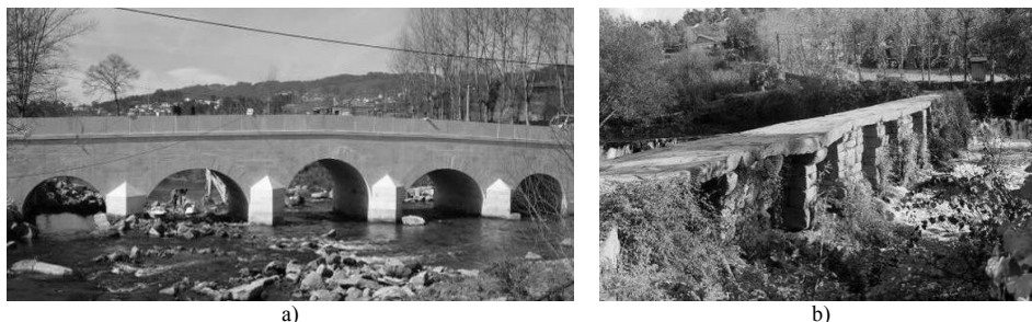
Figure 1 : Vila Fria Bridge. a) new bridge and b) old passage.
