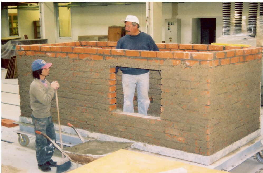
Figure 2: The ACUSTILAB during construction.
