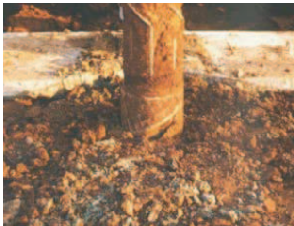
Figure 15 - Omega pile drilling.
