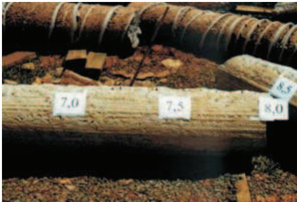
Figure 27 - Shaft view in CFA 2 pile (1 st plan).
