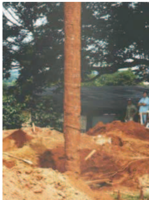
Figure 30 - Soil adherence in shaft of Omega 2 pile.
