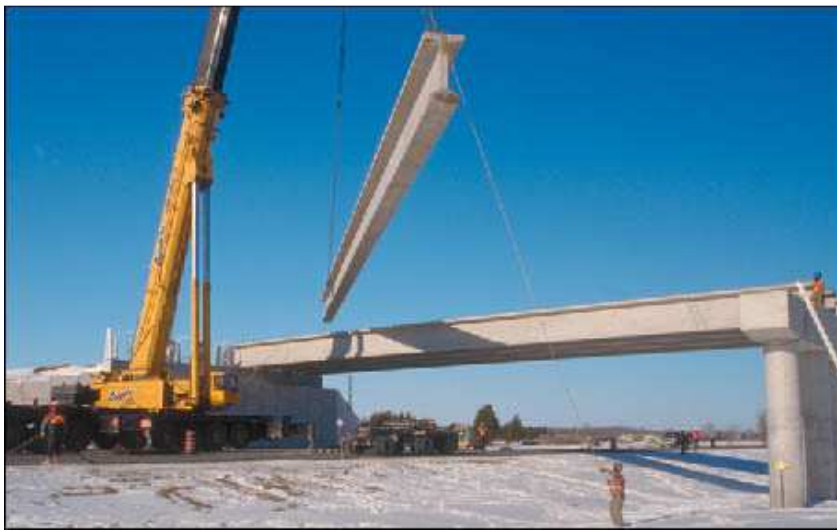
Figure 1-1 – Construction of a bridge deck with precast concrete beams (CPCI 2015).
