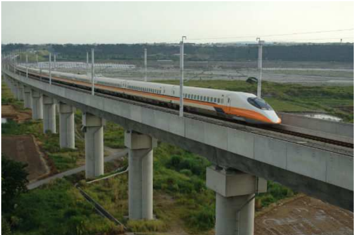
Figure 1-5 – High-speed railway bridge with precast beams (Taiwan 2015).
