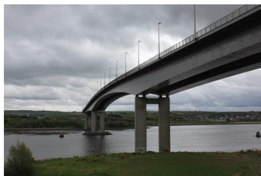
Fig. 2.16 – Ponte Foyle ( moireosullivan.com )
