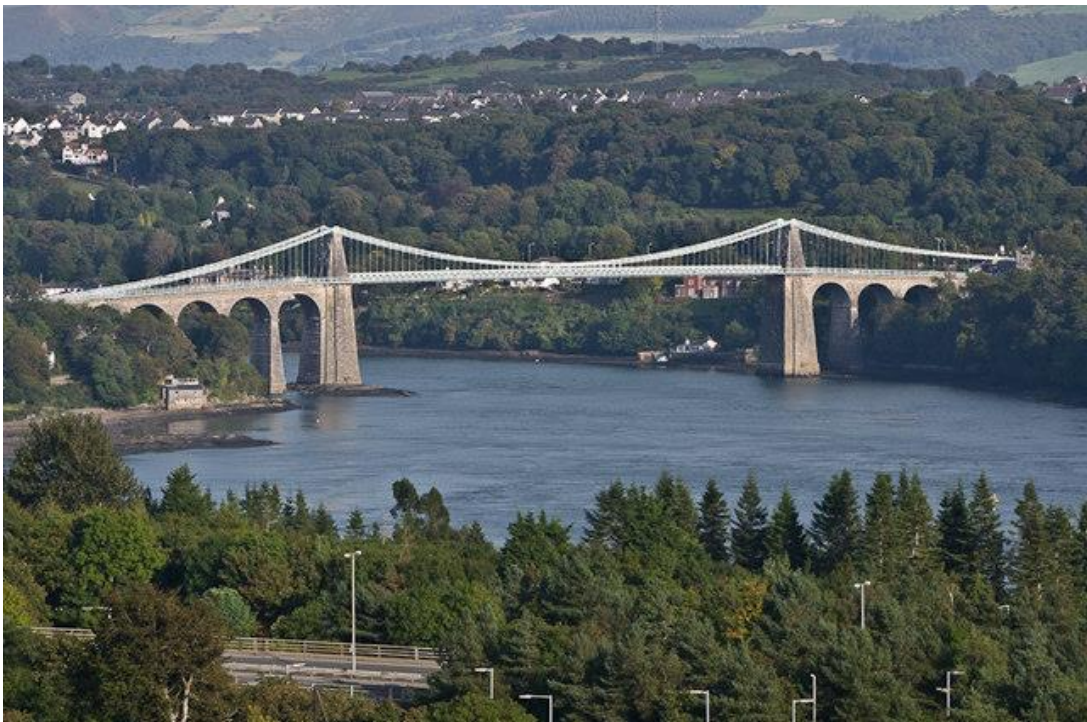
Fig. 2.9 – Ponte suspensa de Menai ( www.geograph.org.uk )
