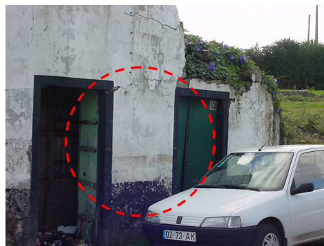
Fig. 1. Building from where the wall was removed.
