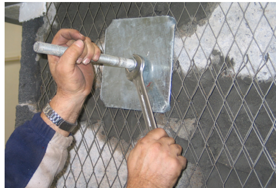
Fig. 20. Reinforcing technique: metallic net and steel rods.
