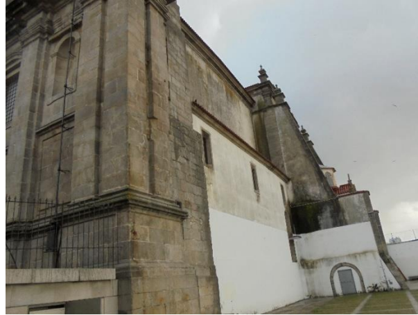
Figure 41. Buttresses at the West zone of the São Lourenço Church.
