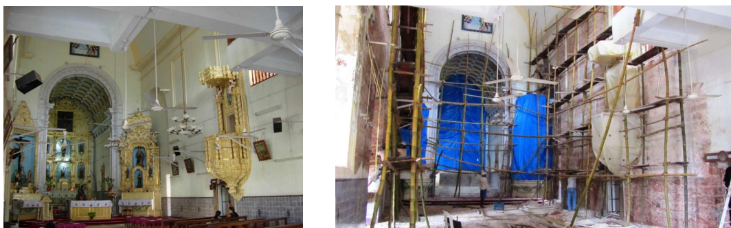
Figure 4: Comparison of the interior of the church before and during restoration.
