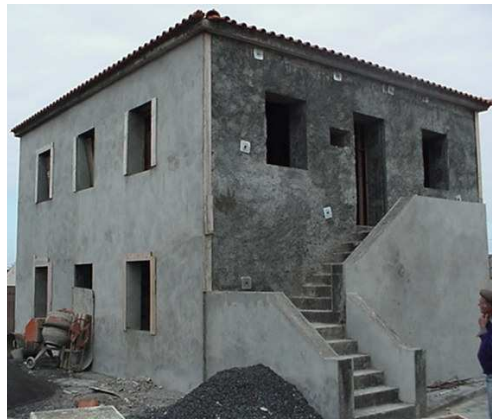
Fig. 15 – Semi-rural house strengthened and partially plastered
