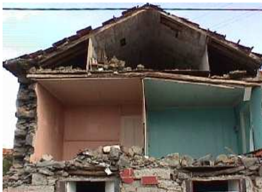
Fig. 4 – Aspect of the building's interior
