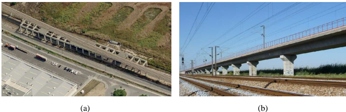
Figure 6.1 - Alverca viaduct: (a) frame area (Fernandes, 2010) and (b) ramp (Malveiro et al., 2013).
