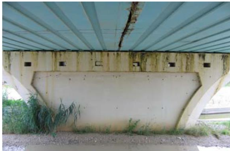
Figure 4.2 – Detail of the longitudinal expansion joint.
