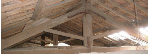
Figure 5. Timber roof structure. António Carneiro building, XX century (1916), Porto.
