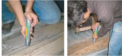
Figure 11. Pilodyn used in a timber floor. António Carneiro building, XX century (1916), Porto.
