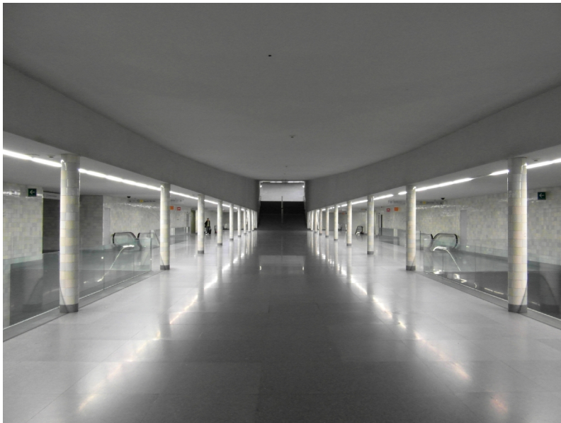
Figure 42 - Porto São Bento Metro station [187]
