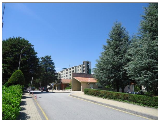
Fig. IV.10 – Vista do Hospital (2012)
