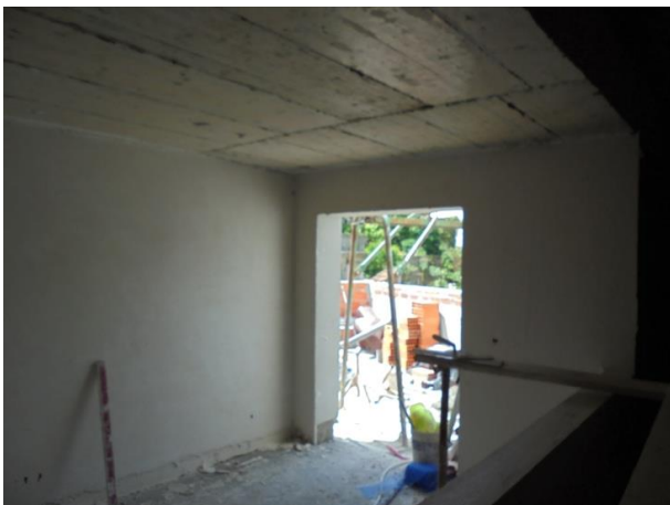
Fig. 3.24 - Reboco interior
