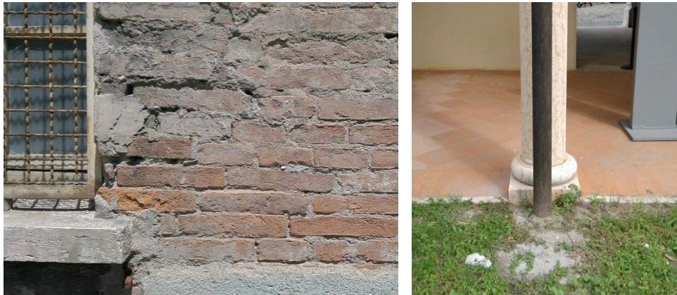
Fig 4.5 – Exterior wall from Diocesan Museum (left); Downspouts in the cloister (right).
