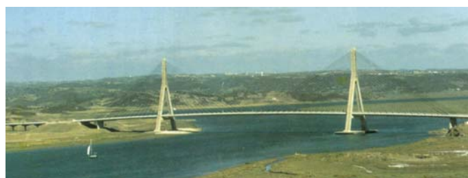
Figure 1. View of Guadiana Bridge (Cândio Martins, 1992).
