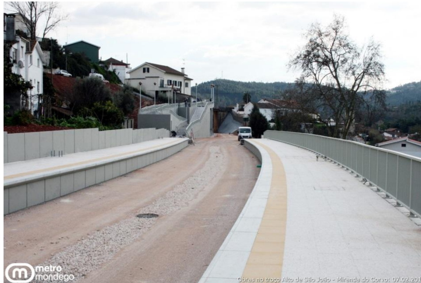
Fig.6.2 – Works made in the Lousã Line [60]
