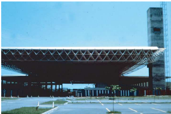
Figure 2.6: International Congress Centre of Rio de Janeiro at Brazil [15]
