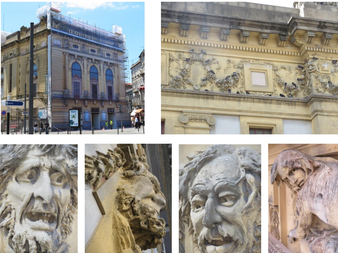
Figure 2 – Façades and reinforced concrete decorative elements of the São João National Theatre.
