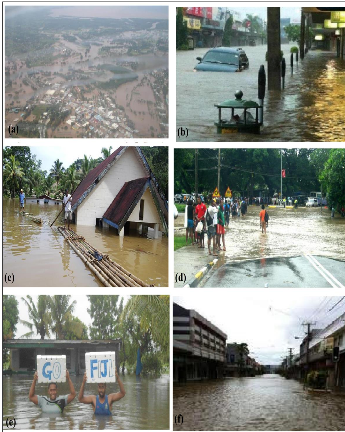
Figure 6 The January 2009 flood caused major infrastructural damage in the western parts of Viti Levu (a) An aerial view of a inundated Nadi town (b) Main road Nadi town submerged in water (c) Villagers located near the Nadi river and tributaries flooded (d) A roundabout on the main road submerged in flood waters (e) Flood waters reach waist high in some areas as shown up two men cheering for Fiji (f) Shops are forced to shut down businesses when flood waters inundate the town during the 2009 flood. (Source: GoogleImages)
