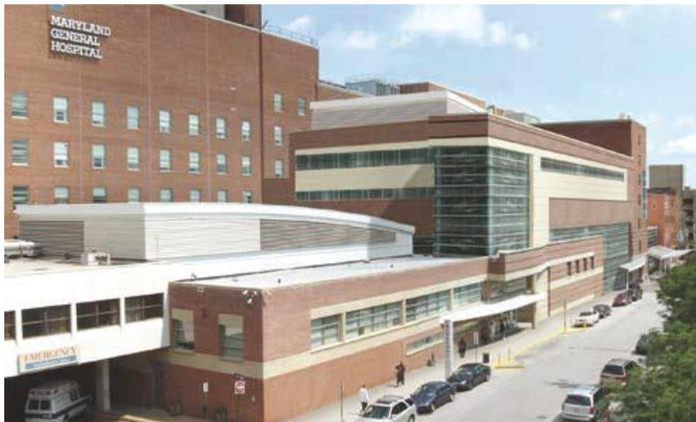
Figure 4.10 - Maryland General Hospital, Baltimore, Maryland [27]
