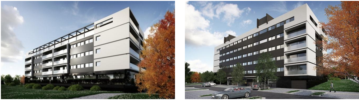
Figure 4.4 – West (at left) and East (at right) building facades (Prumocerto, 2015).
